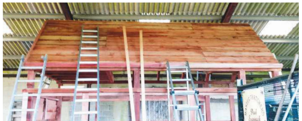
...then the roofing boards
